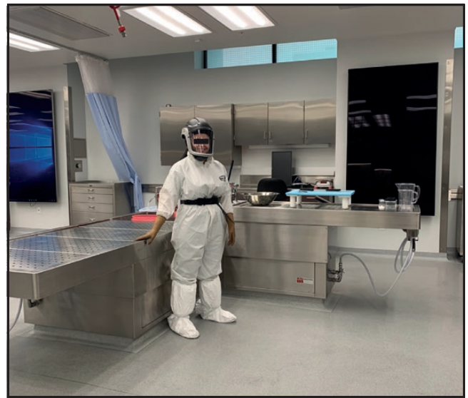
Image 1 A pathology technician in complete autopsy attire. Behind her is an example of the reverse airflow tables at the Oklahoma Office of the Chief Medical Examiner autopsy stations. The main autopsy suite is equipped with 8 identical stations. Suspected coronavirus disease 2019 (COVID-19) autopsies are performed in an isolation room equipped with two identical stations.
